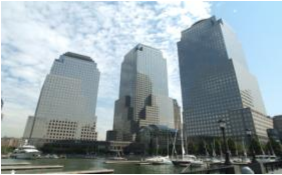
World Financial Center, New York Four tower office complex with over 8 M sq. ft
