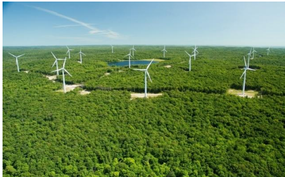
Prince Wind Farm, Ontario One of Canada's largest wind farms with 126 wind turbines and 189 MW of installed capacity
