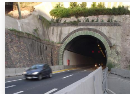
Tunel San Cristobal ("TSC"), Chile
