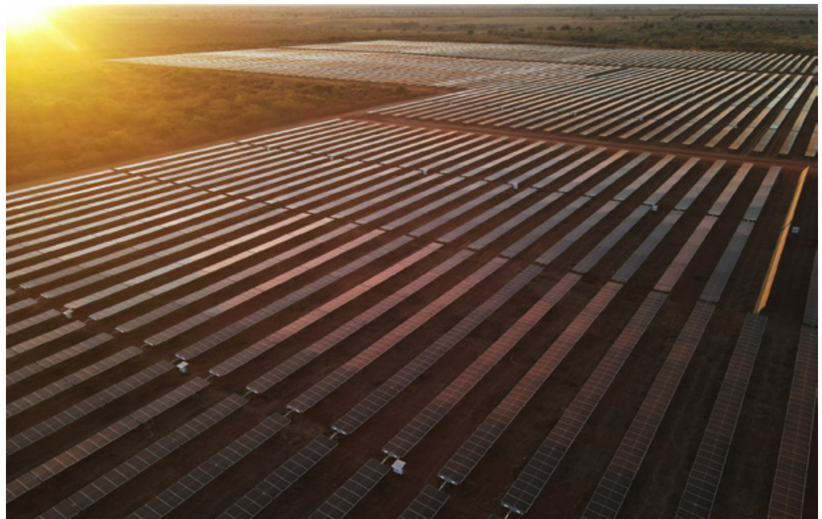
Janaúba Solar Complex, in the countryside of Minas Gerais
