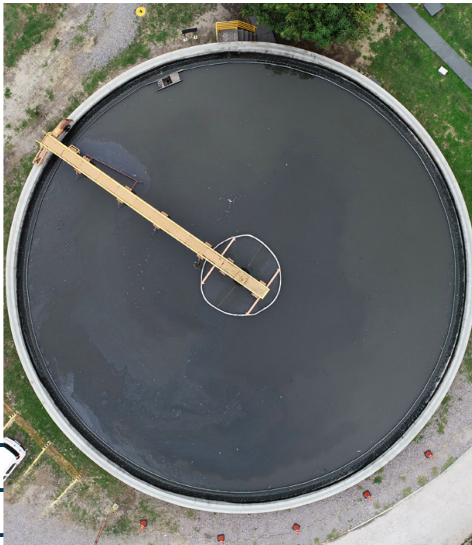
BRK wastewater treatment plant
