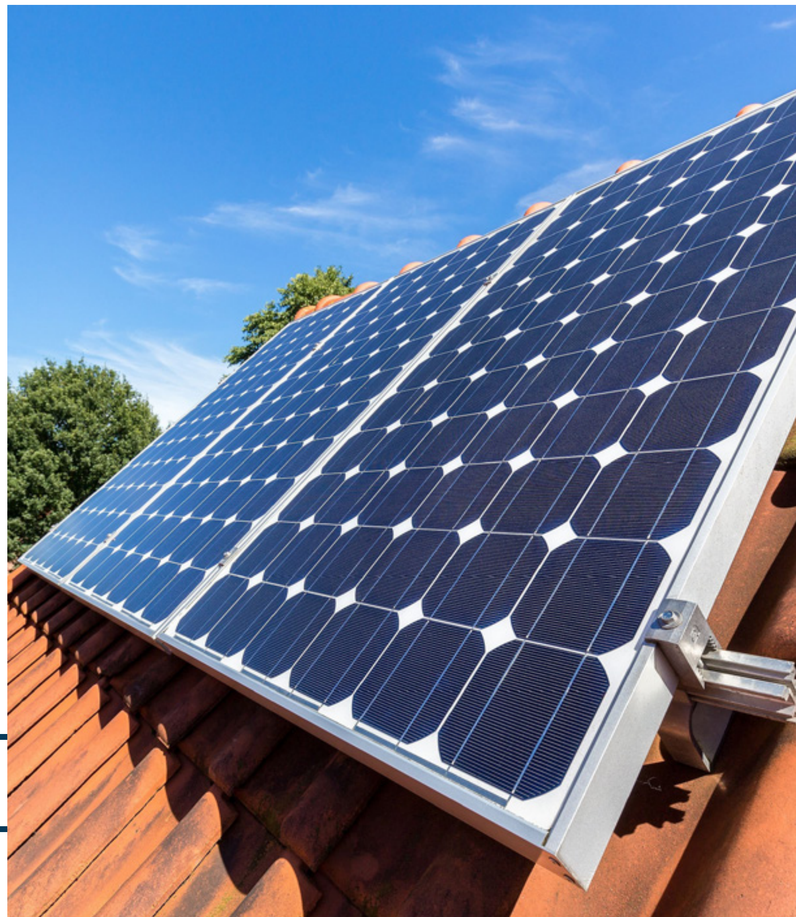
Residential solar panel installation
