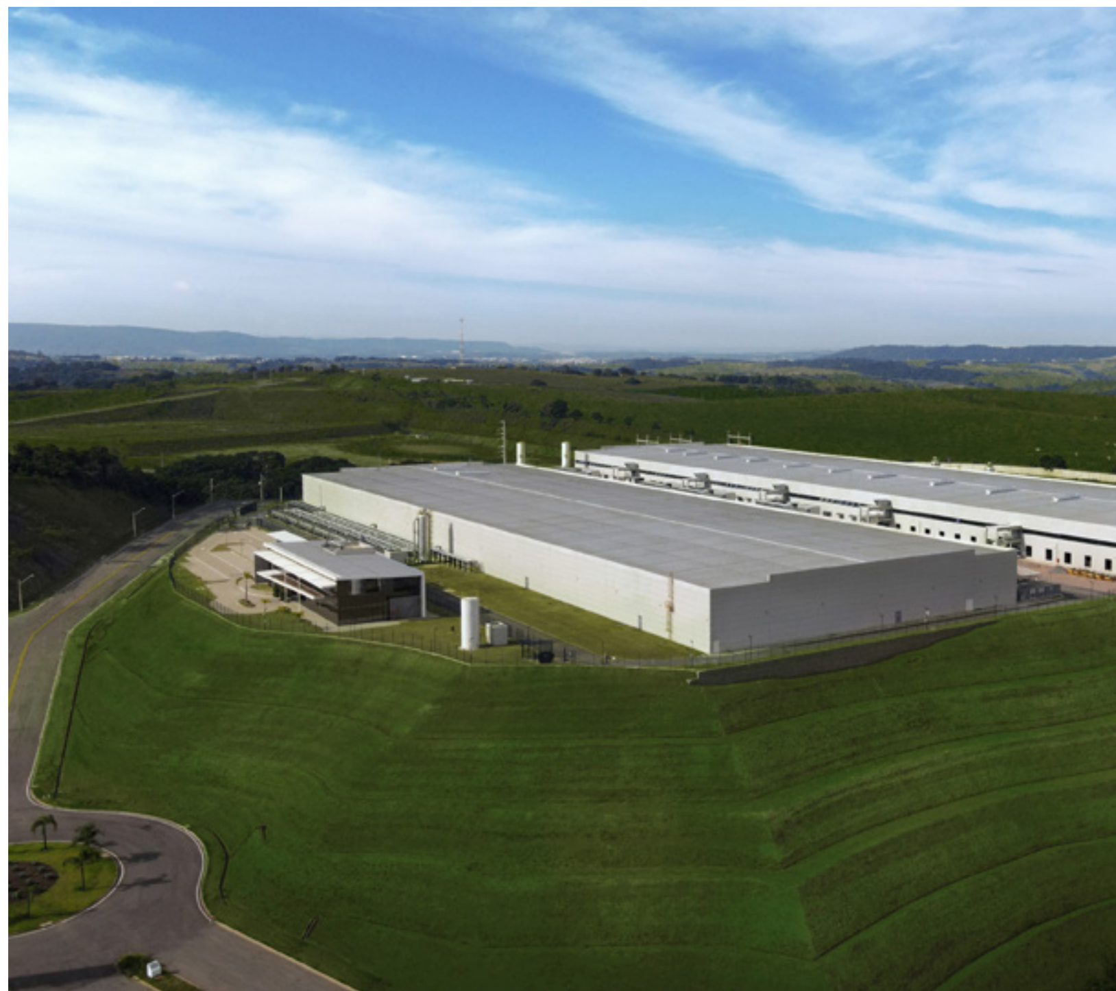
Ascenty Data Center in the countryside of São Paulo
