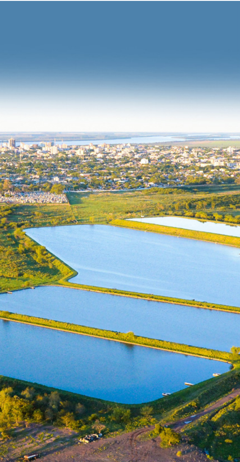
BRK water treatment plant in Goiás
